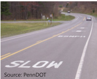
Source: PennDOT These pavement markings remind approaching drivers of the speed limit and notify them of the impending intersection.
