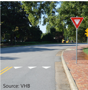
A YIELD sign controls right turns along this skewed intersection approach.
