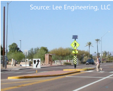
The refuge island allows pedestrians to make this multilane crossing in two stages.
