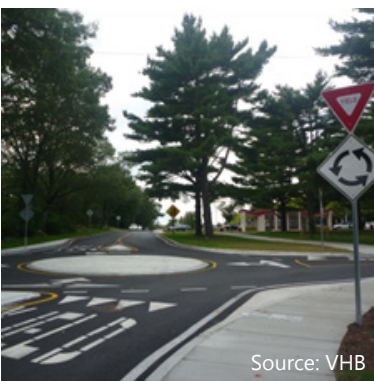
A YIELD sign and supplemental yield line and YIELD pavement marking control each approach to this mini-roundabout.
