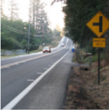
These speed reduction pavement markings are installed with a Side Road sign.
