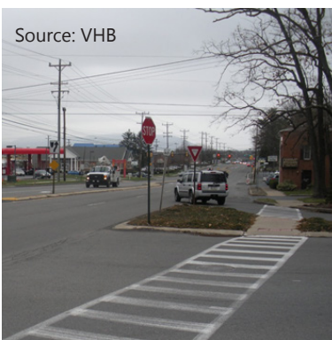
Pedestrian crossing this minor road approach can take refuge in the channelizing island.
